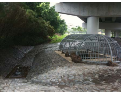
(j) Stormwater overflow drain near York's Hollow, Herston.
