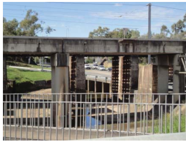
(b) Rocky Waterholes Creek rail crossing, Sherwood/Fairfield Roads, Rocklea.
