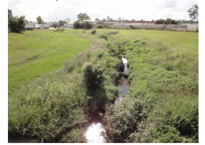
(f) Stable Swamp Creek, Musgrave Road, Salisbury.
